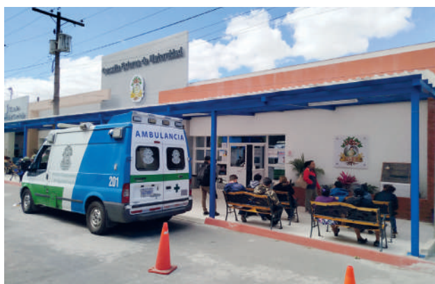
Hospital Gineco Obstetricia.
