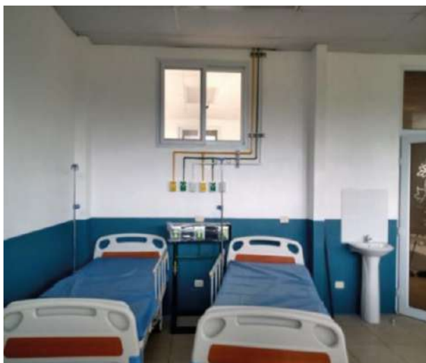
“Hospital de Retalhuleu”
